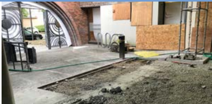
Preparing for new energy-efficient, radiant heat floors. Photo credit: Becky Gibler
